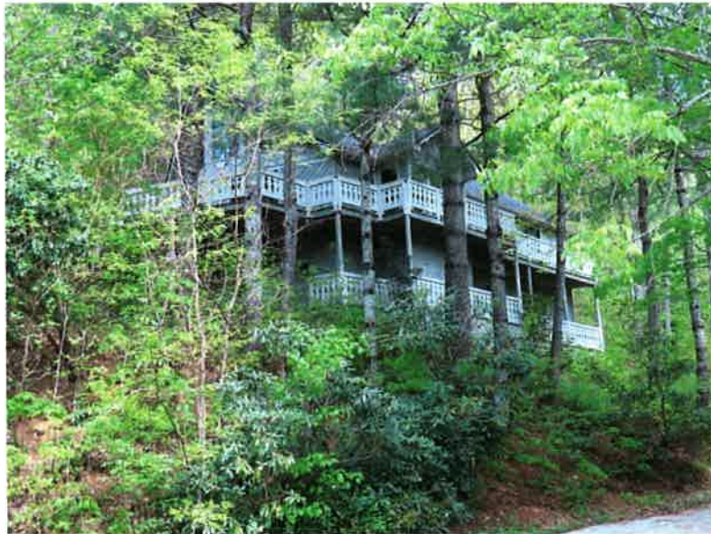
Steep slopes and narrow roadways will hamper firefighting efforts.
